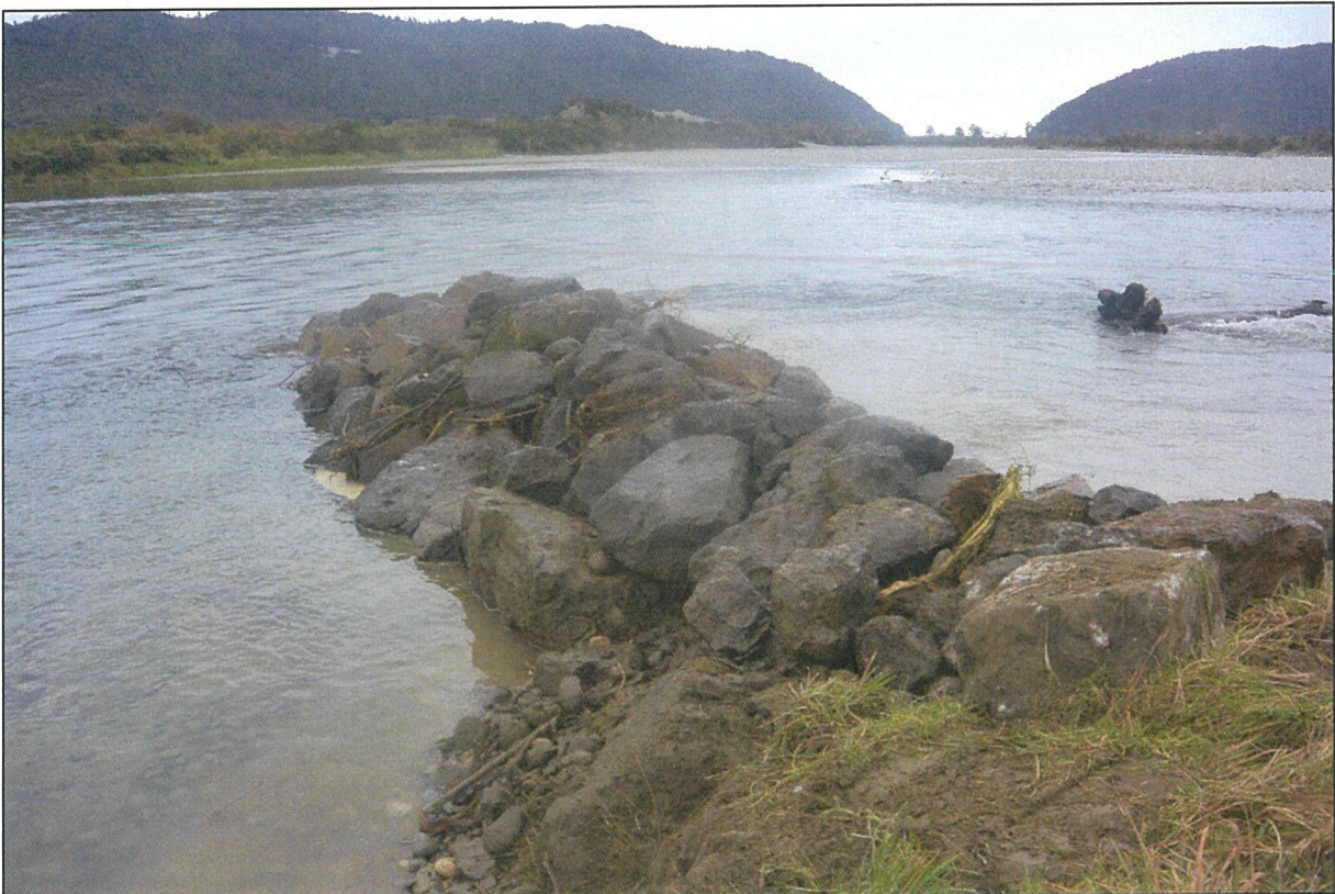
Completed spur, Grey River at Coal Creek
