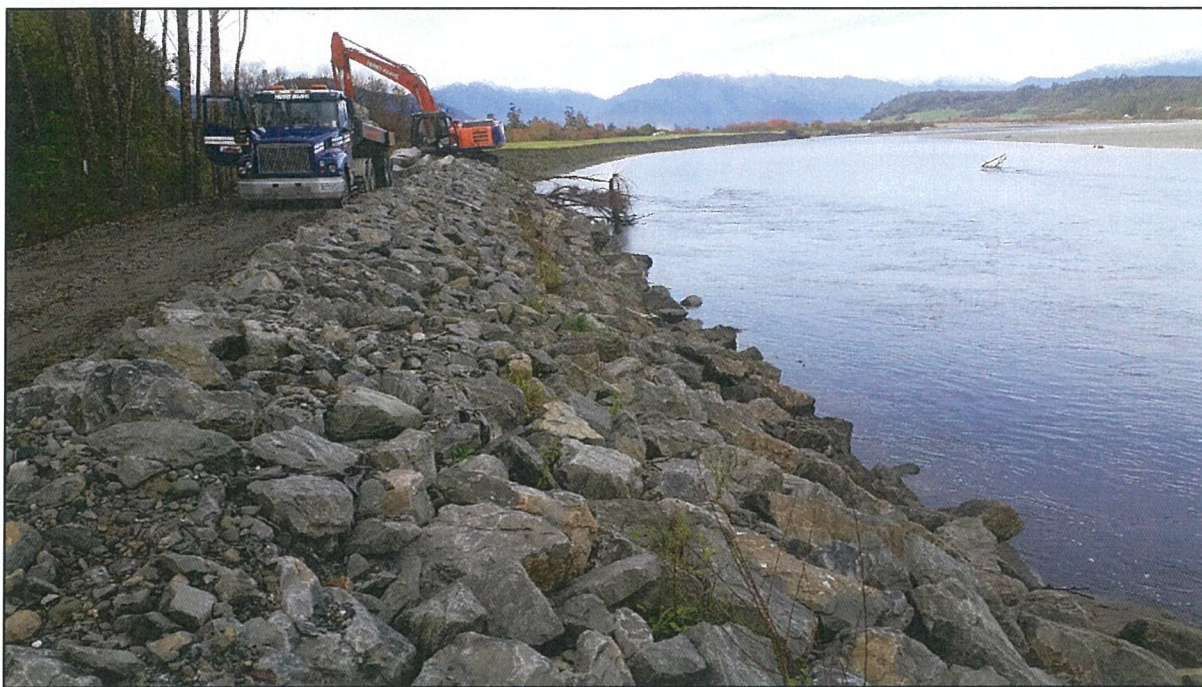
Placement of rock at slumped areas of the rock riprap at Kaniere
